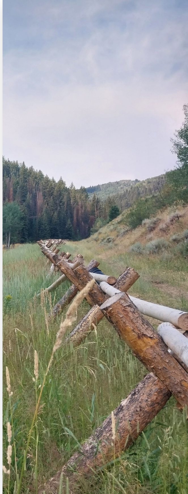
Above: An exclusion fence TU constructed in Big Bear Hollow, designed to keep roaming animals from damaging fragile habitat.
