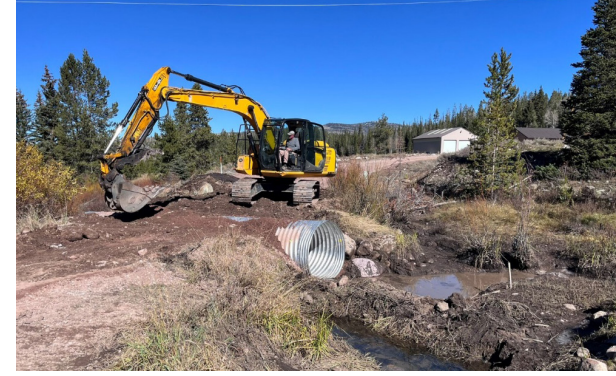
Above: Installing a culvert on Deadman Creek. At right: Boots - and bodies - in the water to install a low tech, process-based structure in the Upper Bear River.
